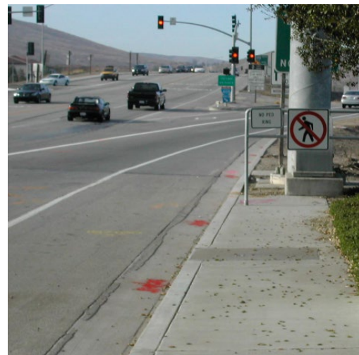
Figure 6. Missing infrastructure as a sidewalk ends at a location with high-speed vehicular traffic. There is a “no ped crossing” sign on display. Source: www.pedbikeimages.org / Barbara Gossett.
